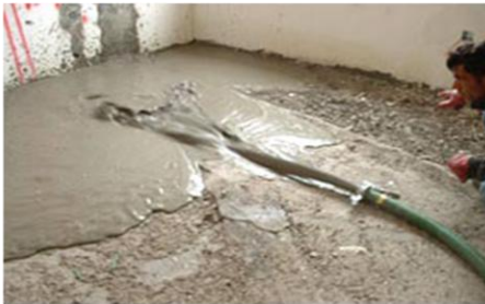
BULLDING FLOOR SCREED
